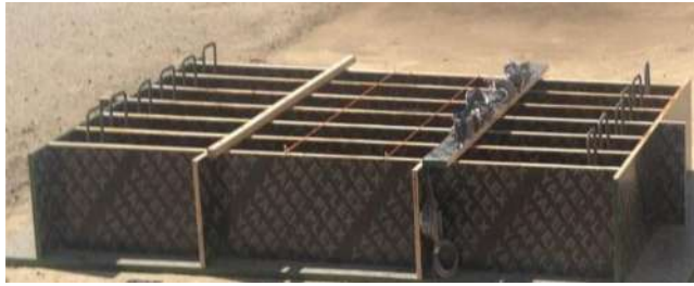
Figure 2. Formwork of the concrete beams.
