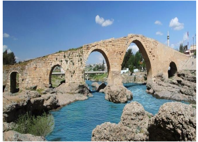
FIG. 1. THE VIEW OF THE DALAL BRIDGE.
