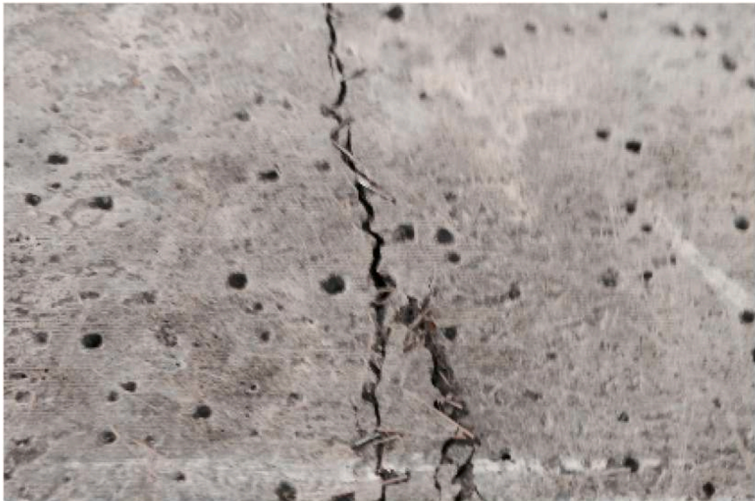
Fig. 6. View of UHPC containing both MSF and HSF.
