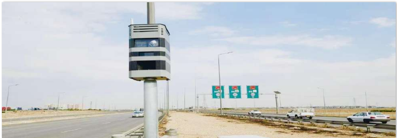
Fig.1 ERBIL-120m street with a point-to-point camera.
