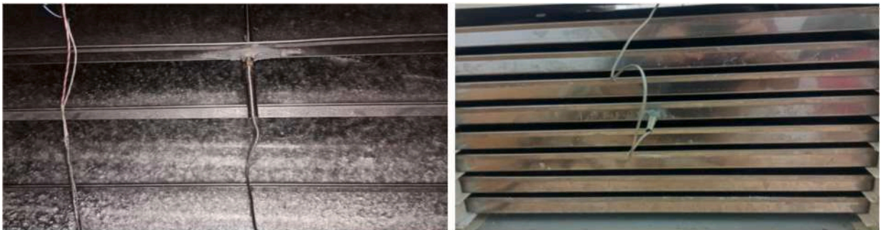
Fig. 9. PCM panels and air channels.
