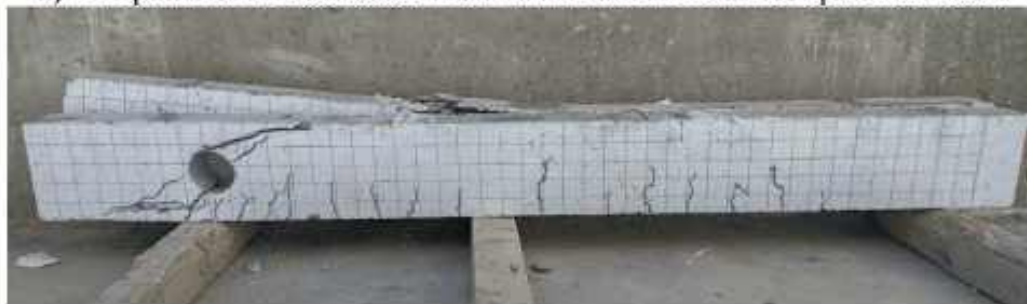
b) The patterns of crack observed and the failure mode for specimen SBLs.
