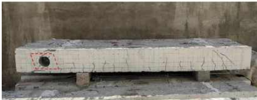
h) The patterns of crack observed and the mode of failure for specimen DBLSP10.
