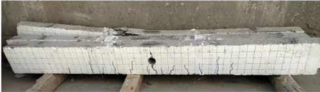
e) The patterns of crack observed and the mode of failure for specimen SBSF.
