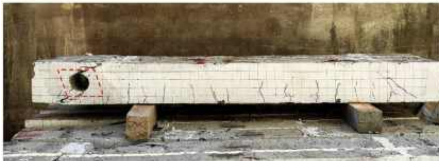
g) The patterns of crack observed and the failure mode for specimen DBLSP8.
