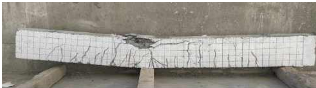
a) The patterns of crack observed and the failure mode for specimen SCB.
