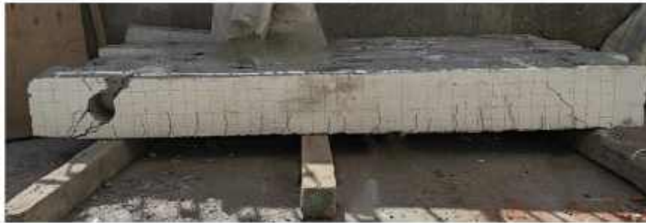
b) The patterns of crack observed and the failure mode for specimen DBLS.
