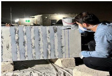
d) A layer of epoxy on the concrete surface.
