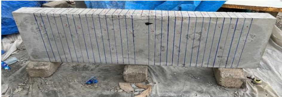
a) Mark the location of CFRP
