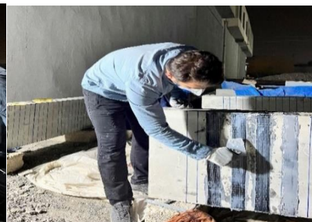
e) Placing the CFRP over the concrete.
